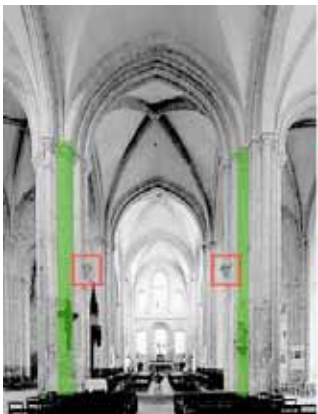
Etampes Notre-Dame with similar isolated capitals in the entry to the choir, (a-) level, marked with red square. Centre, our model of Etampes with suggested timber element between these capitals. Right, Saint-Denis south narthex entry into nave, two capitals shaded blue with similar possibilities (Moulin, Fig. 59).
