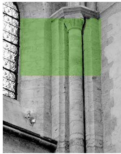
Capitals and supporting shafts on the eastern wall in the choir (c+). Green marks the courses that are bonded into the adjacent windows.
