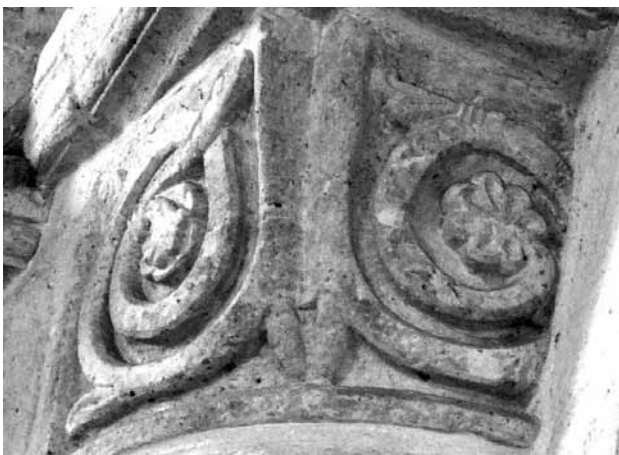
Capital in the EN1(c+) crossing pier
