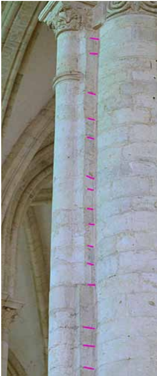
EN1 and ES1 piers with junctions between the pilaster and the drum marked where the coursing appears to be continuous.
