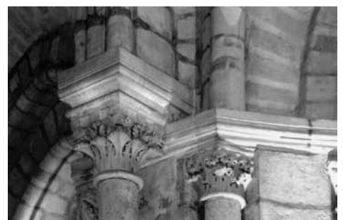
Impost over shaft higher than over windows
