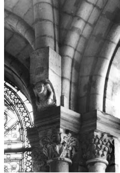
Corbel over wall shafts to support ribs
