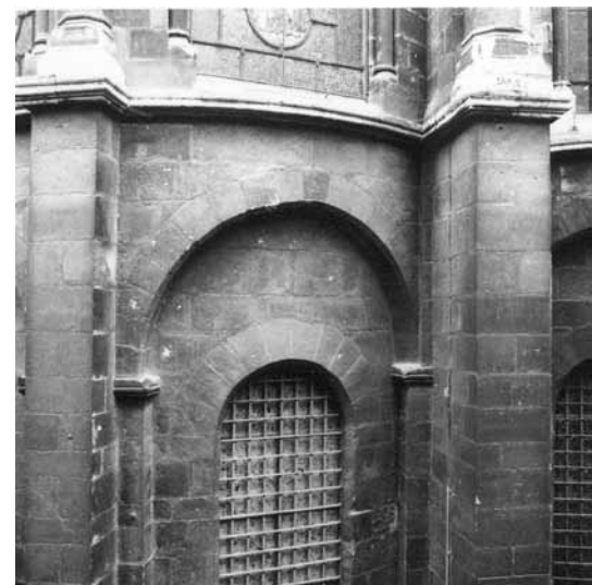
Keystone to relieving arch over crypt windows
