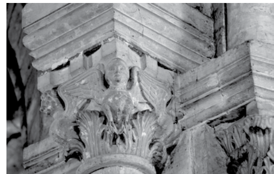
Enchancre in the upper part of shaft capitals, in COGA this design is linked to Notre-Dame aisles from '45 and Bougival crossing in '36.
