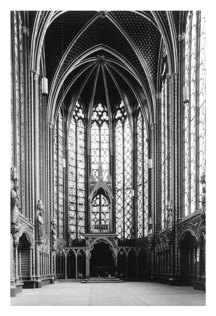
The piers of the upper chapel [r1] are laid out to a different system The "g-g" span is 340mm more than "f-f" in the lower, and forms the proportion with the bay of  $3:\varphi$ . This cannot be derived from simple subdivisions, but only through a geometric figure. It is not hard to do, but the process is geometric while in the lower chapel the process is mainly numeric.
