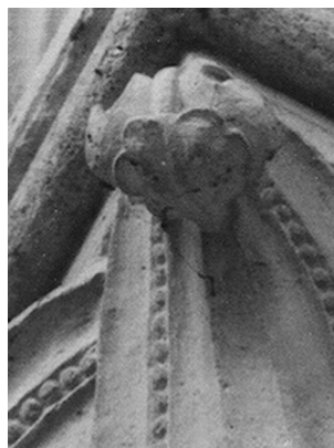
Soissons south aisle
