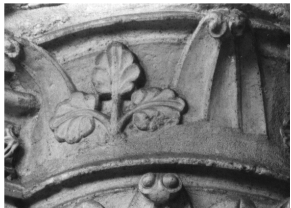
Saint-Quentin ambulatory piers
