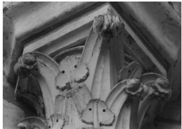
Saint-Quentin ambulatory walls
