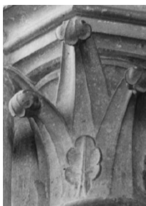
Soissons south aisle
