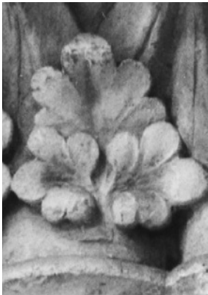
Châlons cathedral nave
