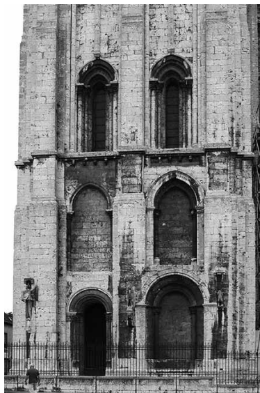
South facade of south tower, "door" on the left
