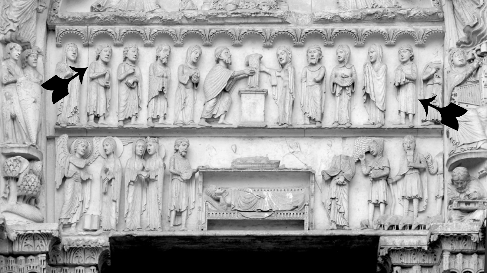
Two lintels in the south, with the joints of the figures that were added to the upper lintel
