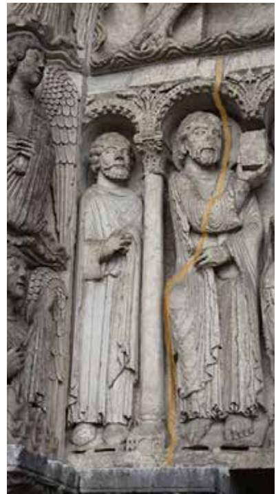
North end of lintel, arch over statue disappears behind architrave, approximate location of crack.
