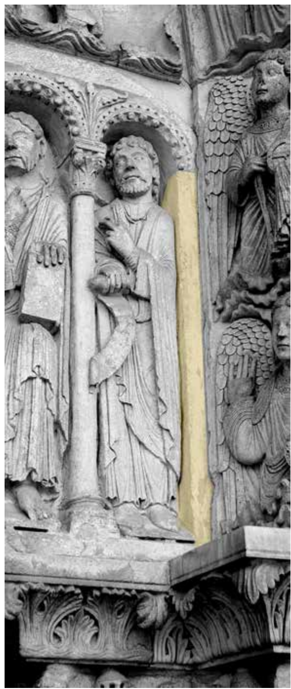
Central door, lintel with inserted frame on the right
