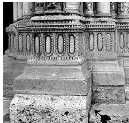
Vertical sides to lowest course under pilasters
