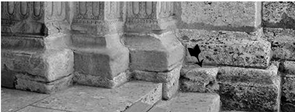
South door plinths against the tower and the small nib that marks the junction between campaigns G and H.
