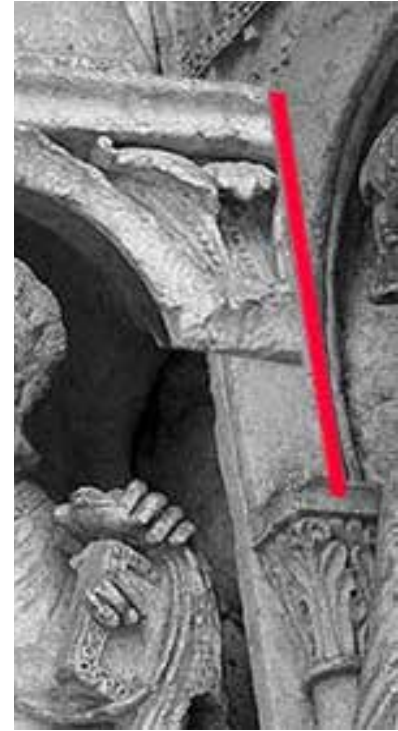
Detail with matching extension to arch
