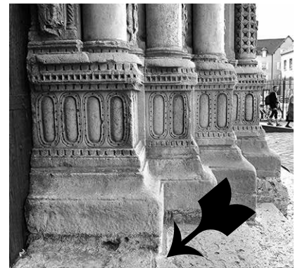
South side north door with upstand.
