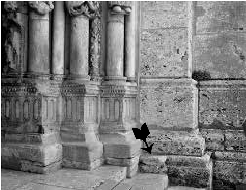
South door plinths sit the tower and the small nib that marks the junction between campaigns G and H.
