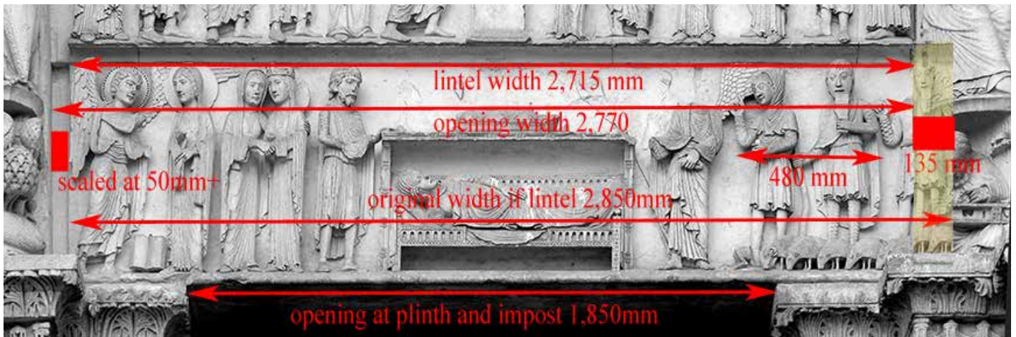
South door, lower lintel with dimensions in millimetres.
