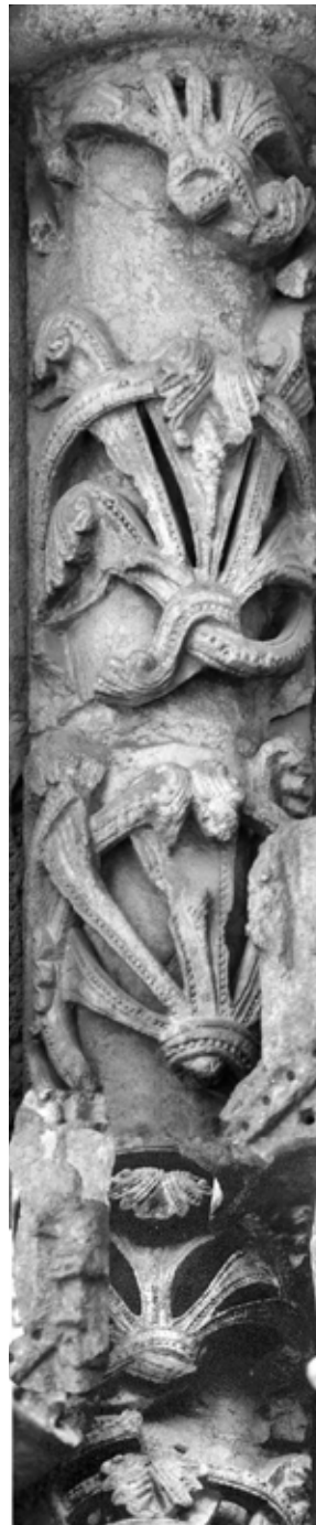
North left nL2t base and top cut off
