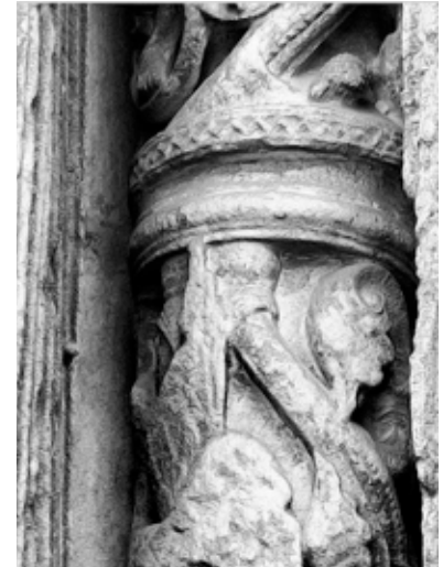
The ring moulds that terminate the uncut shafts
