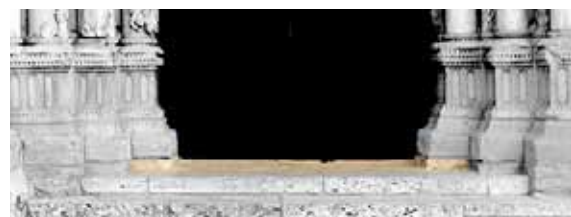
North door threshold with upstands for the plinths.
