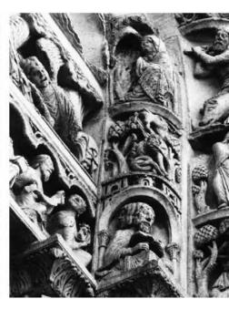
On the left the bottom is set in from the top N [b], so it is flush with the face of the lower lintel J [r1]. The set back of the lower projection from the edge of the archivolt with the personification of April is clearly shown. On the right there is no set back between the upper projection and the lower, both of which line up with the lower lintel M-K [r].
