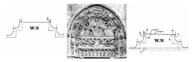
the distance between the lower lintel and the outer edges of the imposts over the historiated capitals is the same on both sides. This means that the imposts are also out of line, I, and so are the jambs and embrasure figures under them. Once again, the erection gangs may have been responsible, for when they placed the lintel, they may have set it evenly over the imposts without checking their placement against the other doors of the portal.
