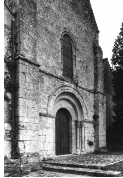
Saint-Martin-de-Bréthencourt west wall
