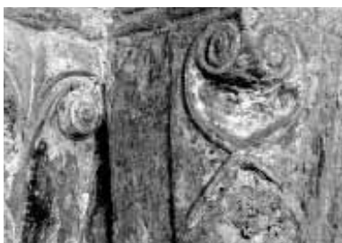
Louvres, Saint-Reuil tower base
