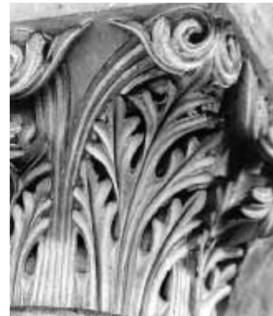
Laon aisle Ne2s(a) corner detail
