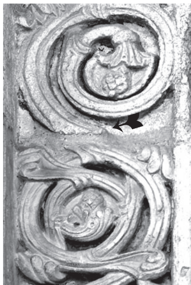
Joint between jamb panels Bourges south porch
