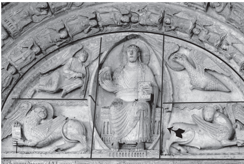
Bourges south portal, tympanum with joints marked
