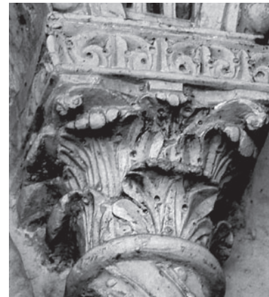
Bourges south portal lintel capital
