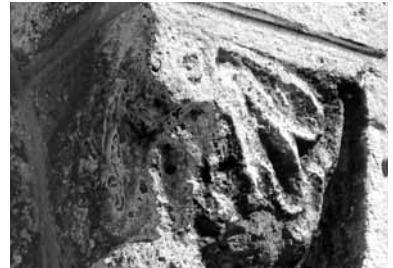
Pont-Saint-Mard west front (aw) 1080
