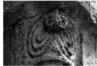
Rhuis tower level 3
