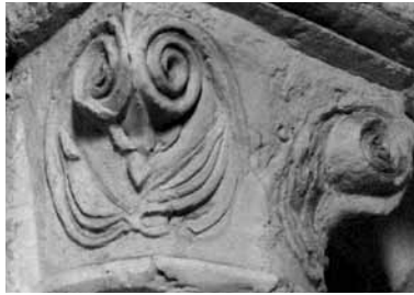
Acy-en-Multien tower base
